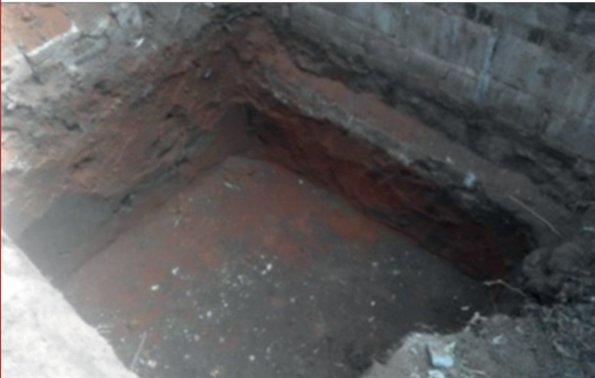
Leach pit hole before lining with bricks, CFHD, 2018
